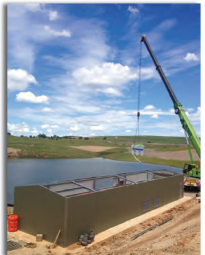
The remote location made for a challenging Installation
